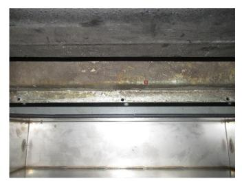
Mark the holes on the bottom of the box from underneath, remove box and drill holes, deburr.
